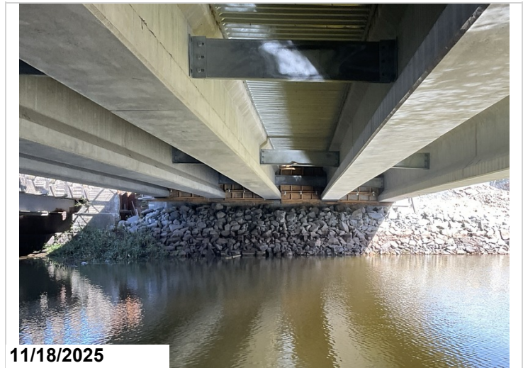
Bent 1: integral abutment overview.
