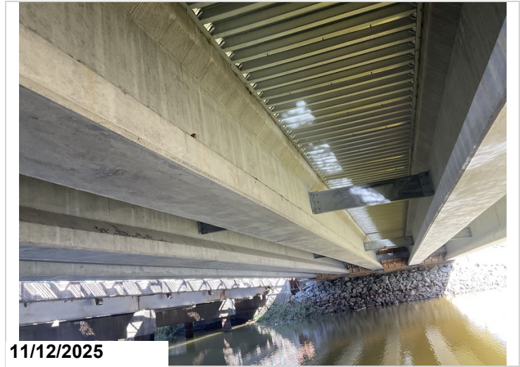
General prestressed concrete girder condition.
