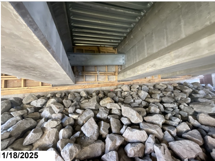
Bent 2: integral abutment overview.
