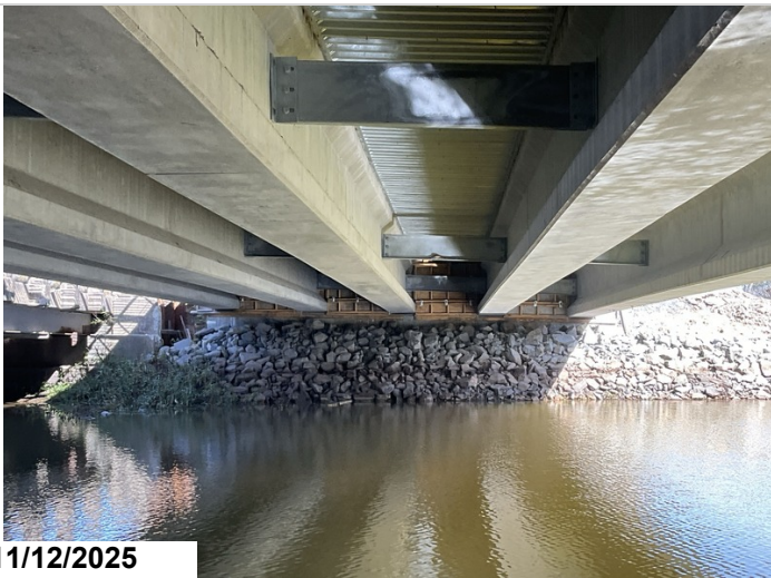
Bent 1: integral abutment overview.
